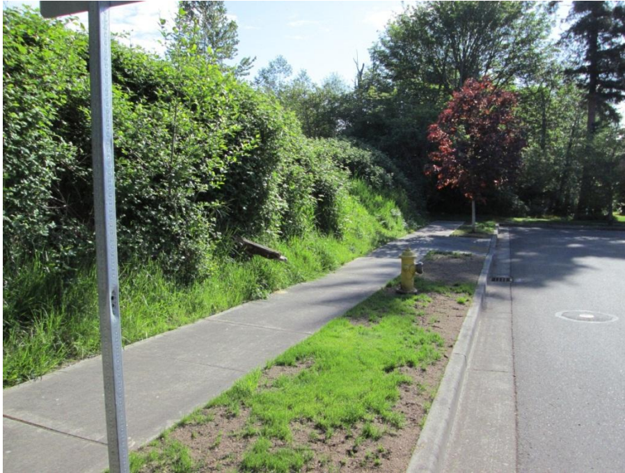
Photo 5: Facing east along southern boundary of site. Runoff from South Basin sheet flows into catch basins within NE 122 nd St.
