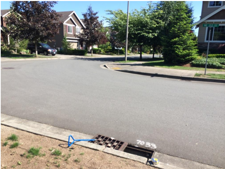
Photo 6: Facing southeast across NE 122 nd St toward 178 th PI NE from the southern boundary of the site. Runoff is conveyed south within 178 th PI NE by 12" pipes.
